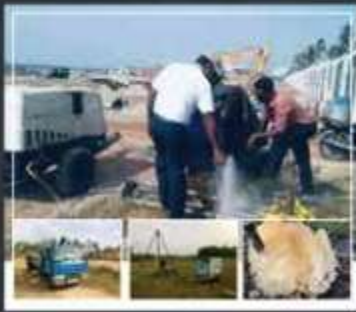
Airport Katunayake 15 Deep Well Project
